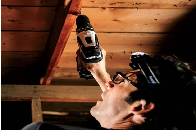
Gambar 6.3 Pengeboran lubang locator
