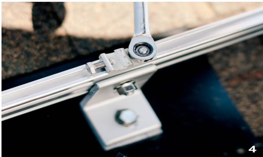
Gambar 6.22 Pasangkan lug grounding
